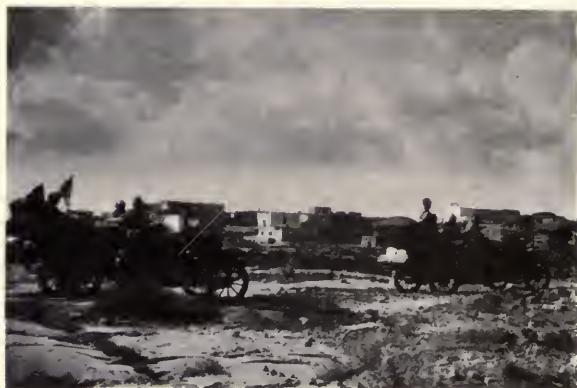
Passing the Pueblo of Laguna, New Mexico. This little Indian republic, with its old church and storied apartment houses, is directly by the path of one of the main transcontinental motor routes
